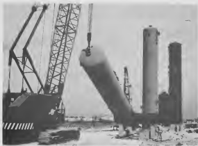
AT THE Baredera industrial site, a heavy-duty crane positions a first-stage absorption tower. The big tower is one of many process units that will make up the Antilles Chemical Company plant. It weighs nearly forty-three tons and stands nearly sixty feet in the air.
